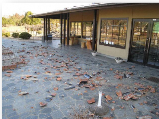
[安達ヶ原ふるさと村瓦崩落]
