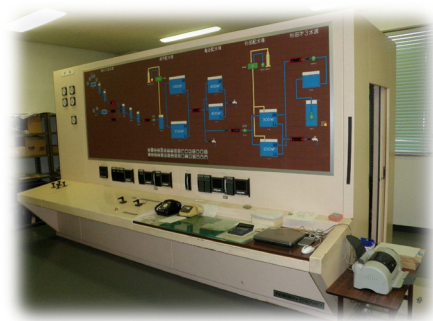
[高平配水場監視室]
