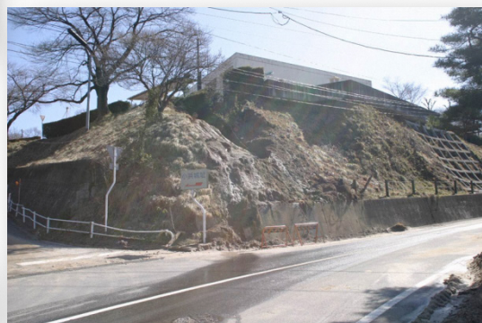
[岩代支所敷地内法面崩落]
