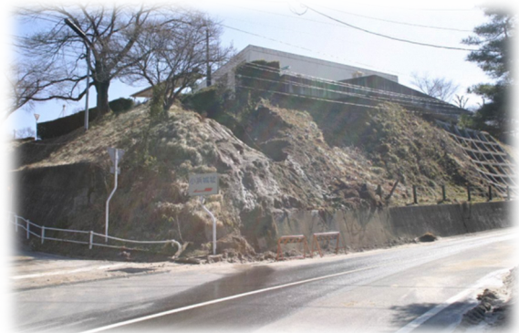
[岩代支所敷地内法面崩落]
