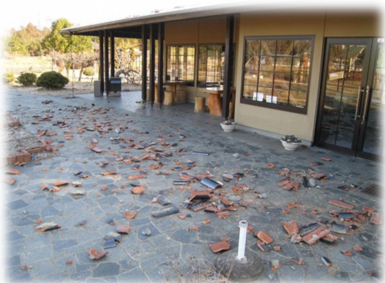
[安達ヶ原ふるさと村瓦崩落]
