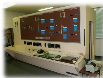
[高平配水場監視室]
